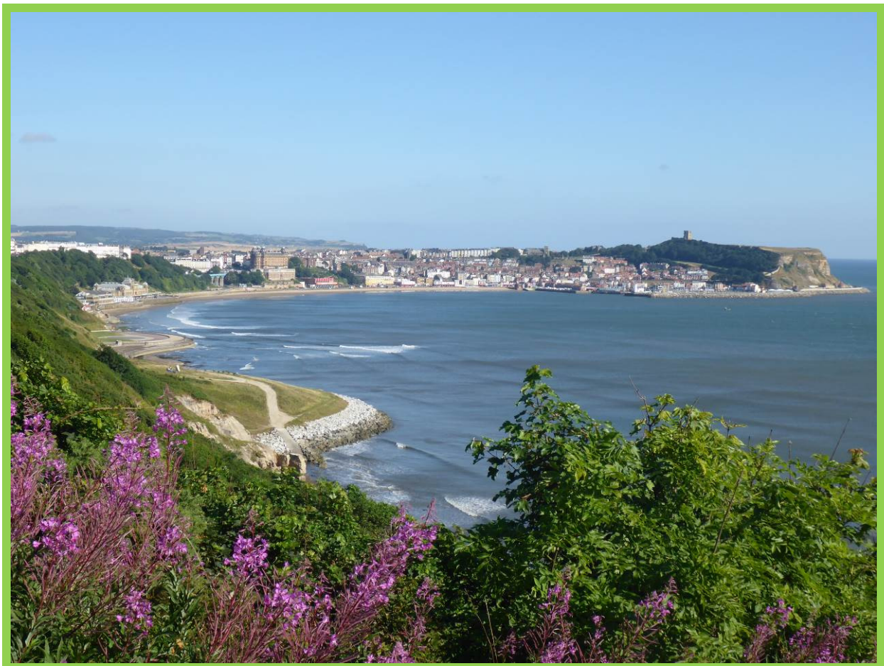
Rock revetment around debris lobe of Holbeck Hall landslide (/1304C01)
