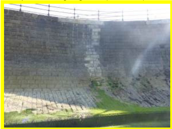
Previous repairs to seawall (/1201C21)
