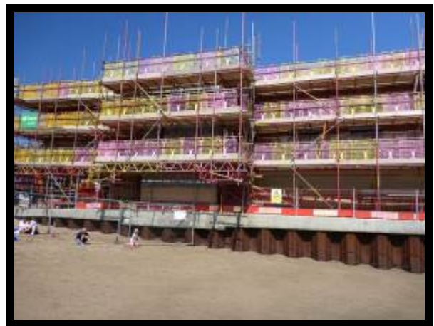
Construction of new RNLI lifeboat station and slipway (/1301C08 & C20)
