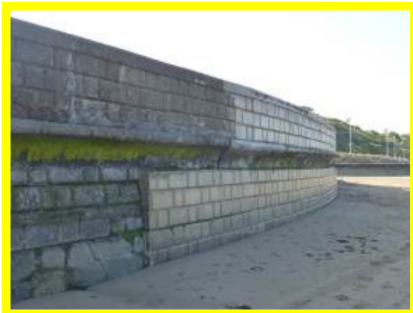
Area of recent repairs to promontory wall (/1201C04)
