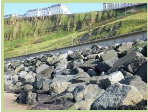
Rock armour revetment and wave return wall (/1202C03)
