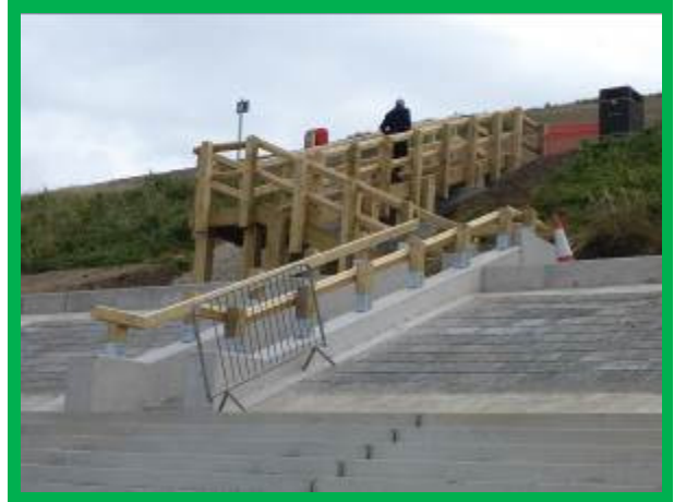
Access steps (\D0702C01)
