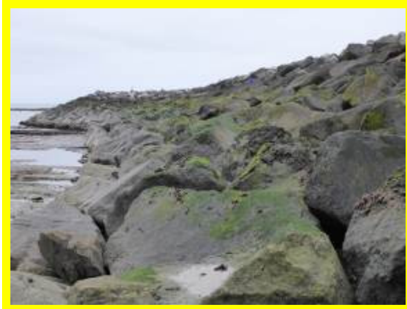
Rock armour revetment on seaward face of North Breakwater (/0402C01)
