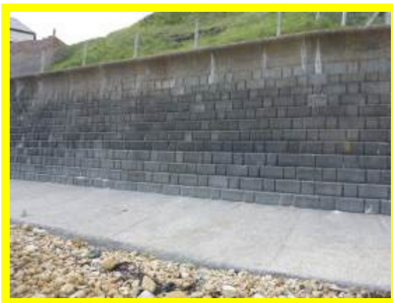
Private sea wall in fair condition (/1402C02)
