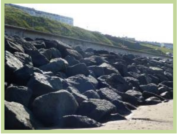
Rock revetment fronting seawall (/1202C01)
