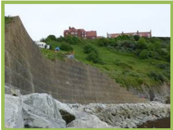
Rock revetment fronting large sea wall (/1003C01)
