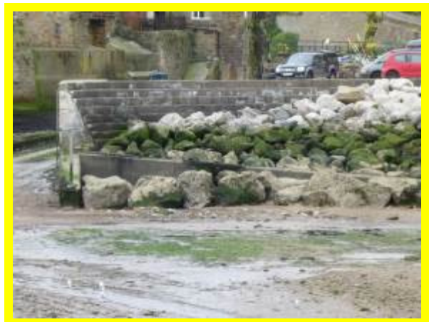
Exposed section of wall south of rock revetment (/0402C02)
