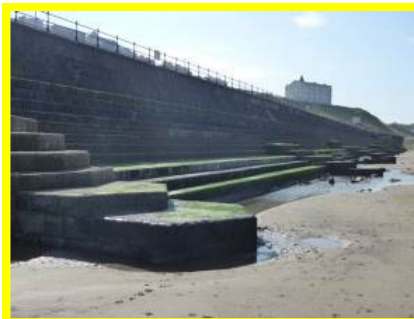
Concrete blockwall wall with buttresses (/1201C08)
