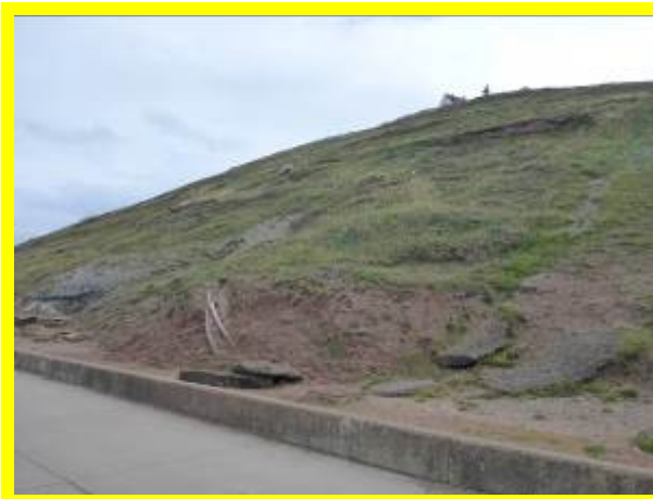
MU11/1 Evidence of slumping in the lower coastal slopes (Locally Active)
