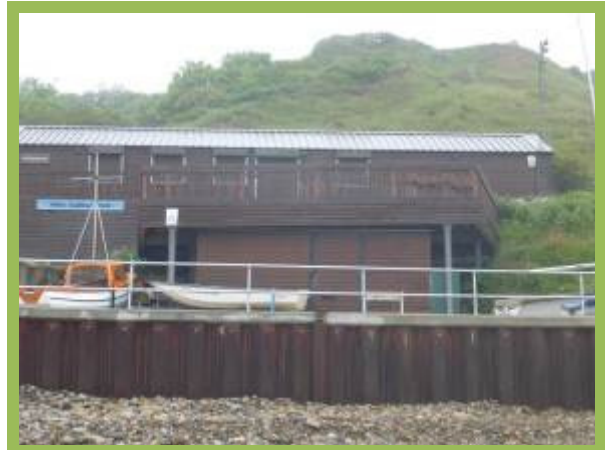
Repaired central section of steel sheet piling as observed in June 2016 (/1601C02)
