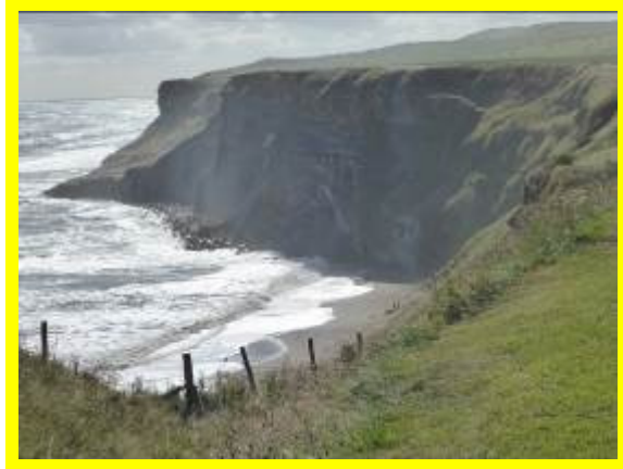
MU13/3 Rockfall at cliffs within Saltwick Bay (Locally Active)
