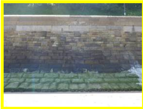
Occasional minor defects but overall fair condition seawall (/1301C26)
