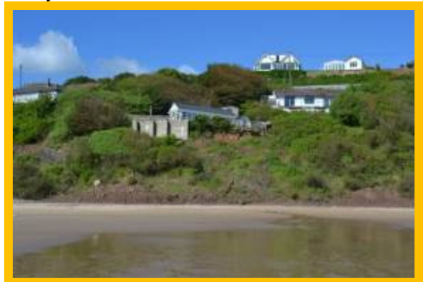
Toe of till cliffs at Flat Cliffs. MU27/AR Partly Active in June 2016
