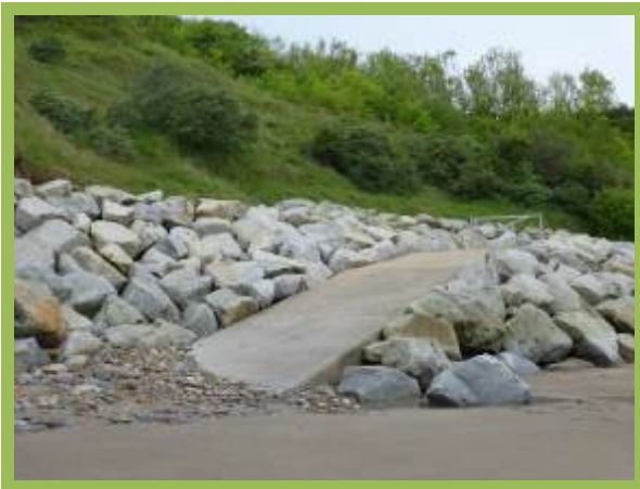
Rock revetment and slipway remain in good condition (/1003C09)
