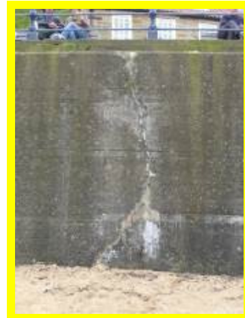
Previous seawall repairs holding well (/0403C01)
