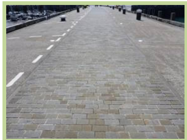
Good condition pier deck on Vincent's Pier (/1301C04)
