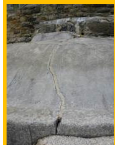
Previous repairs to crack in toe apron are holding well (/0601C06)
