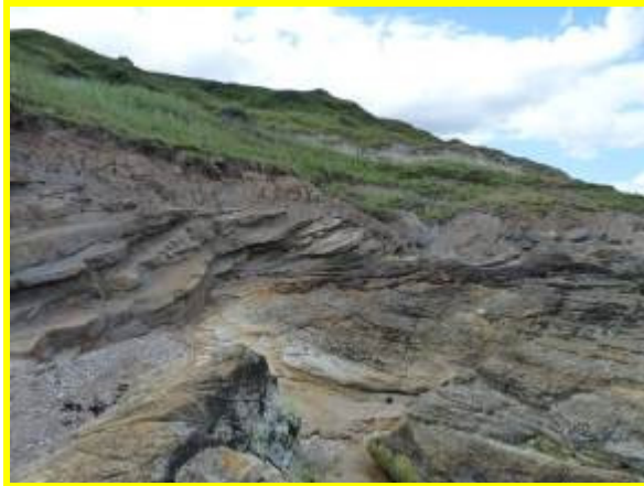
MU23/E Vegetation and localised erosion (Locally Active). August 2014.
