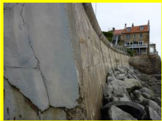
Concrete sea wall generally in fair condition (/1003C10)
