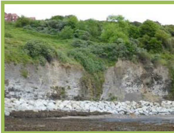
Rock revetment fronting sea cliffs (/1002C02)
