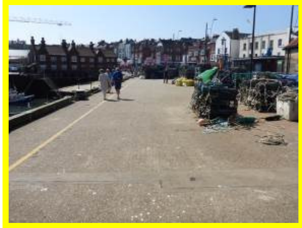
Suspended deck of concrete jetty (/1301C6)
