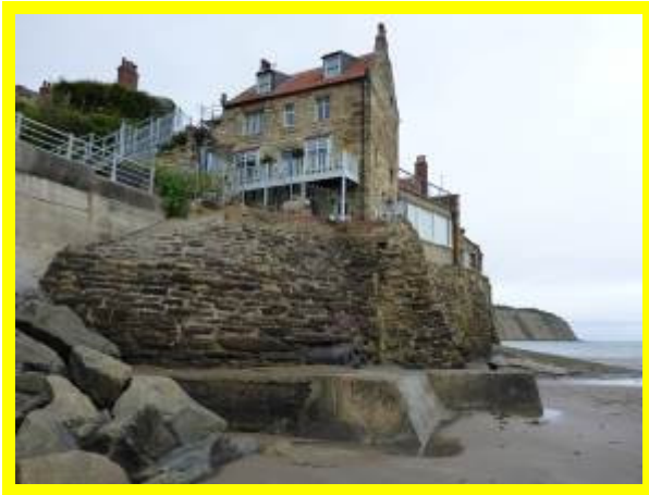
Wall and apron in fair condition but minor maintenance needed (/1003C06)
