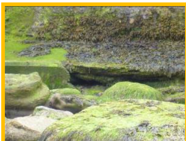
Junction between new concrete toe and original undercut toe (D0802C03)
