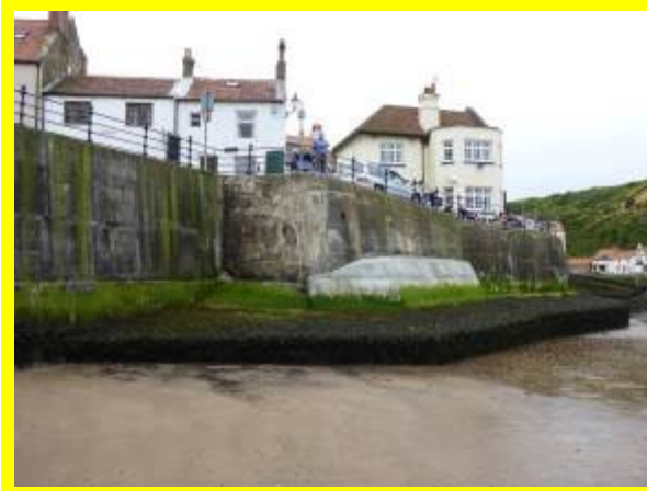
Recent toe berm addition to wall west of Cod & Lobster (/0403C05)
