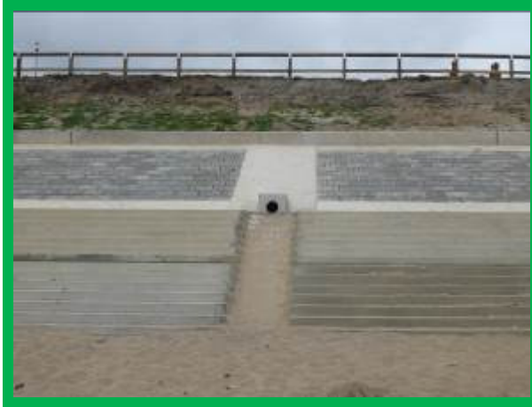
Drainage outfalls and construction ribs (\D0702C01)
