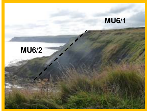
MU6/1 – The eroding shales of the east facing side of Old Nab (Partly Active). The stabilised lobe of material in the background is MU6/2. August 2014.
