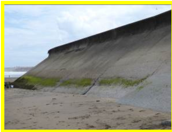
Sandsend car park sea wall (D0701C02)
