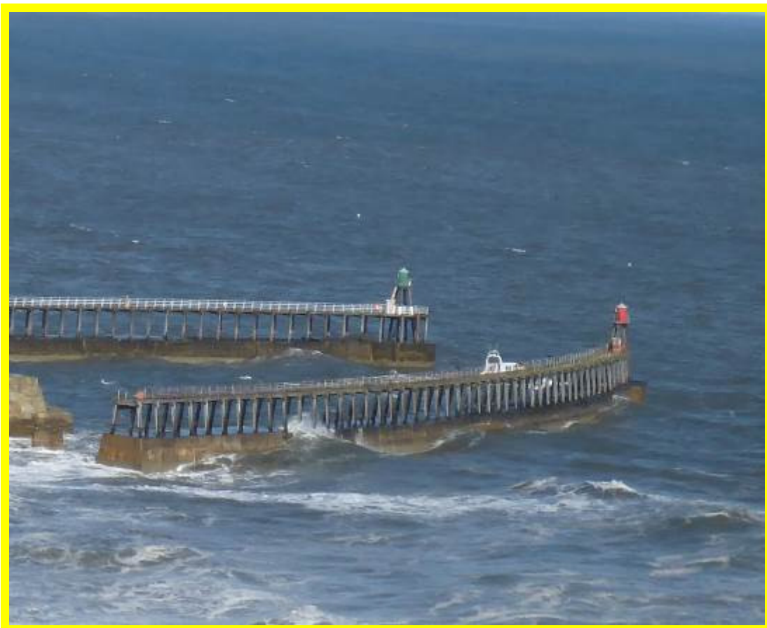
East Pier extension, generally in fair condition (\803C04)
