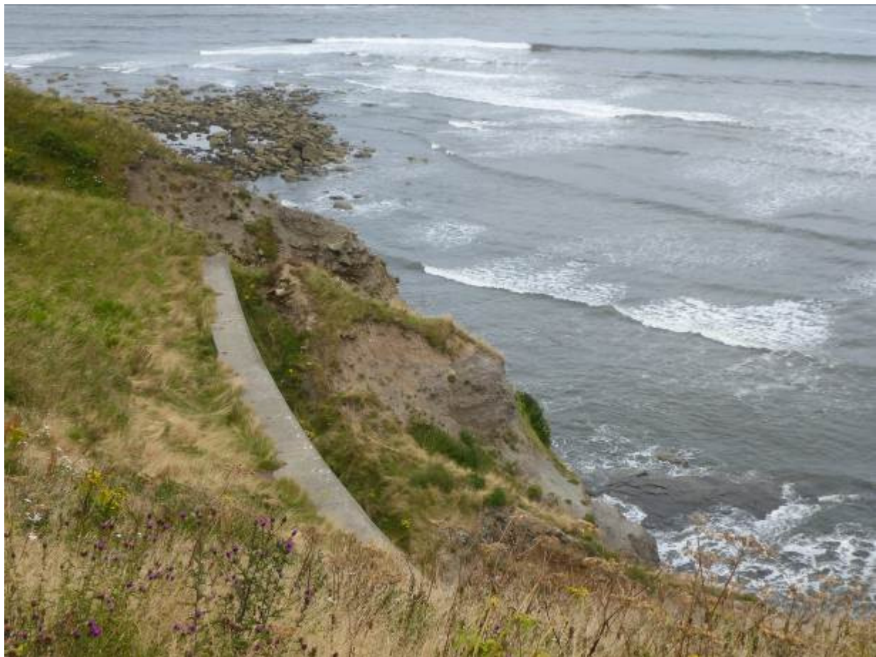
Redundant retaining wall in MU8/14
