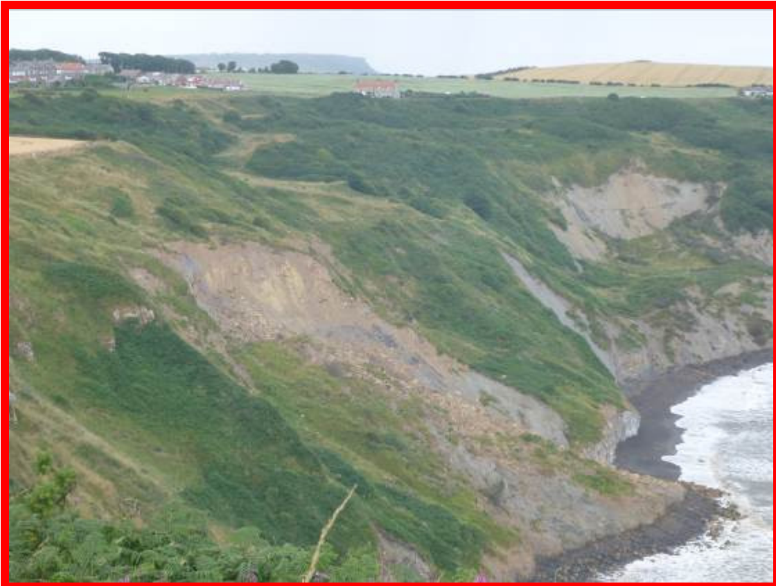
MU6/5 – View of the landslip looking across Port Mulgrave from east to west (Totally Active)
