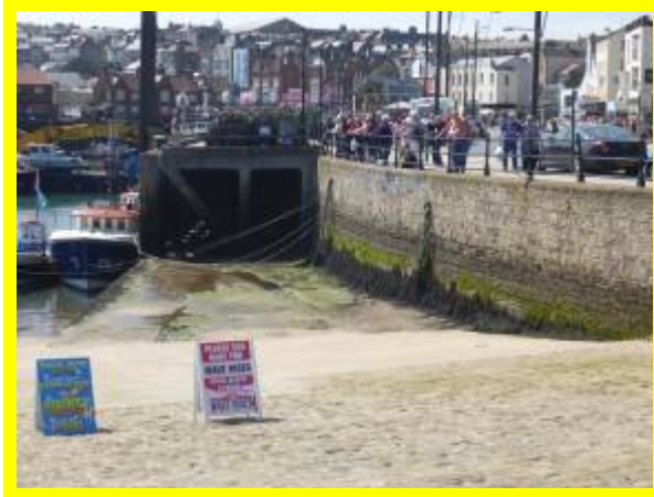
Slipway, quay wall and concrete jetty (/1301C11 and C06)
