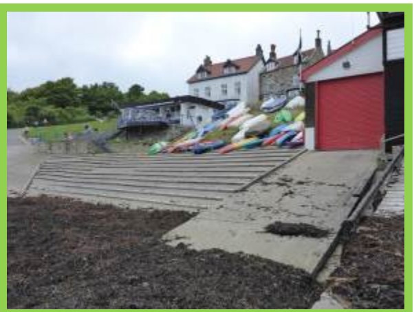
RNLI slipway and adjacent boat storage (/1003C04)
