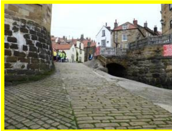
Slipway in fair condition (/1003C05)
