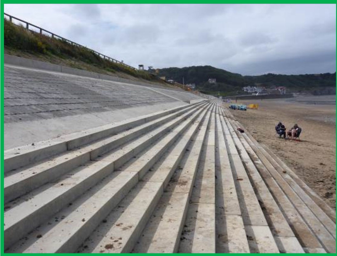
Cross section of coastal defences at Sandsend Road in 'as built' condition showing stepped pre-cast apron and upper Dycel units (\D0702C02)
