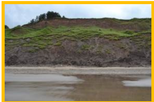
Active till cliffs down to beach level in Robin Hood's Bay. MU17/5 Partly Active in June 2016
