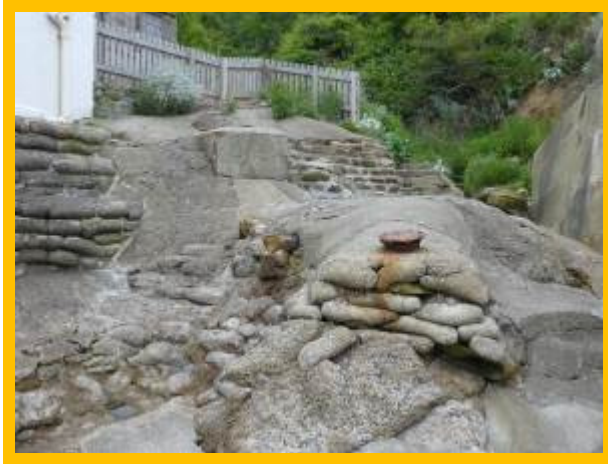
Bagwork wall in front of thatched cottage (/0601C06)
