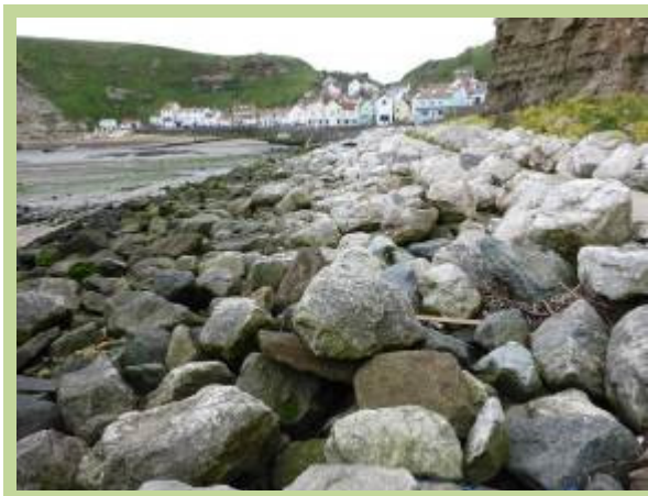
Rock revetment (/0402C02)
