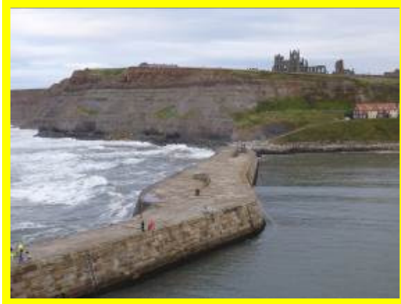
Rock armour protection to toe of Abbey Cliff (\803C06)
