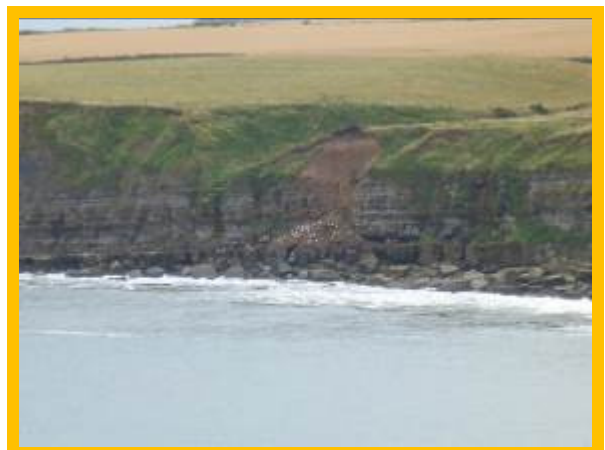
MU19/6 Rockfall on southern side of Cloughton Wyke (Partly Active)
