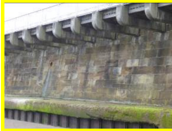
Masonry blockwork sea wall with cantilevered footway (\D0702C04)
