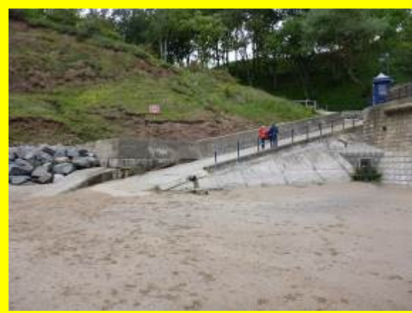
Slipway / access ramp at southern end of Filey Sea Wall (/1602C02)
