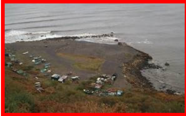
Overview of asset in 2012 (\D0502C01)
