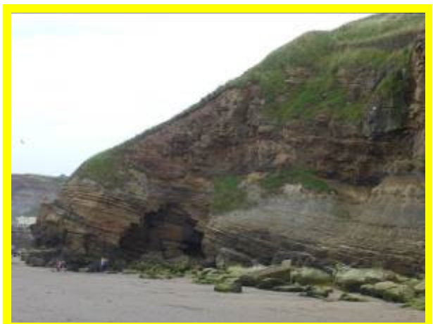
MU11/4 Minor erosion in undefended cliff (Locally Active)
