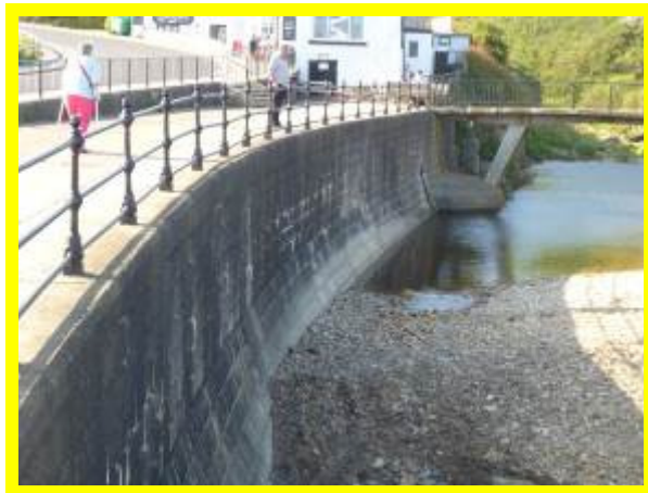
Fair condition seawall at Scalby Beck (/1201C01)
