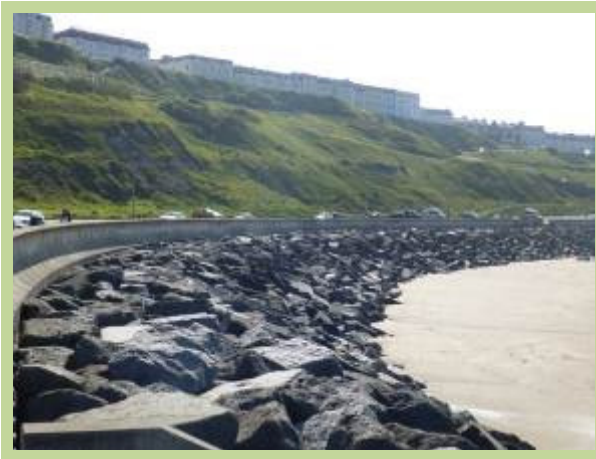
Rock armour revetment and wave return wall (/1202C03)
