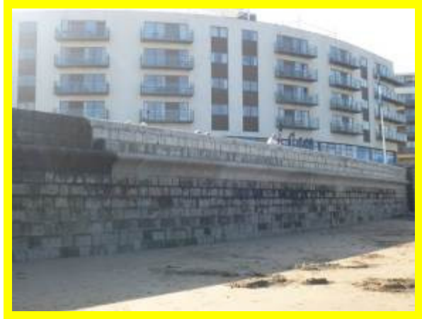
Previous repairs to wall at Peasholm Gap (/1201C19)
