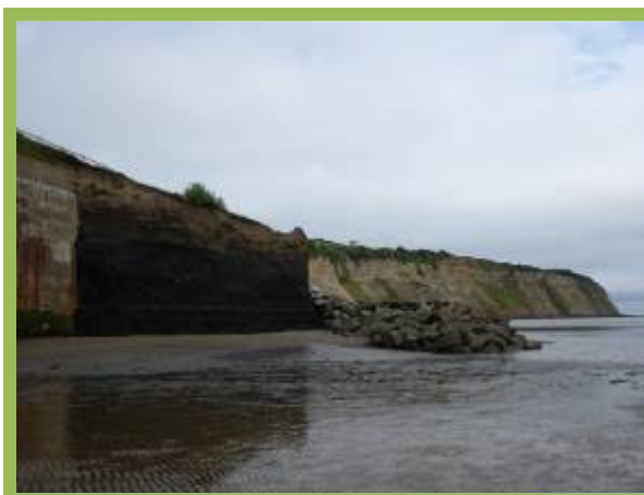
Rock revetment protruding beyond undefended cliffs (/1003C01)
