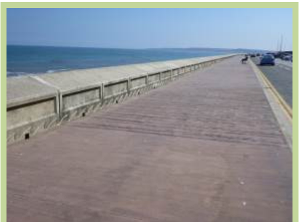
Promenade deck and wave return wall around Castle Headland (/1202C04)
