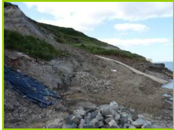
MU23/F Works encountered during the 2014 survey (Inactive). August 2014.
