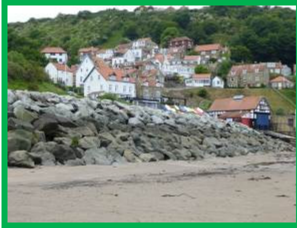
Rock armour revetment (/0602C01)
