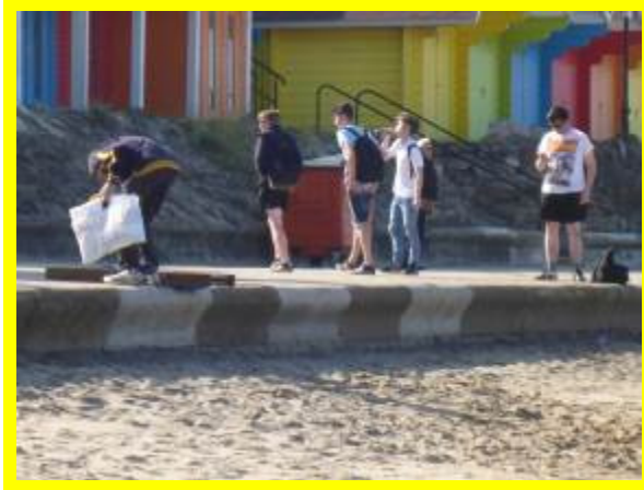
Previous repairs to capping beam at rear of promenade (/1201C05)
