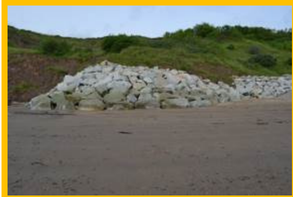
Protected toe of till cliffs in Robin Hood's Bay. MU17/2 (Partly Active in June 2016)
