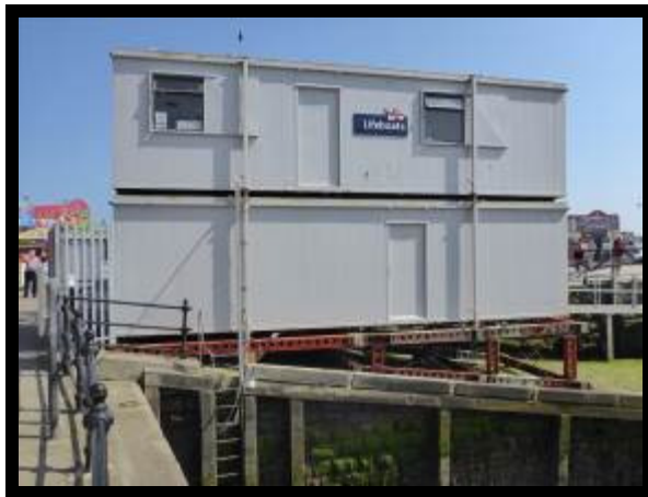
Portable cabins used by the RNLi while a new lifeboat station is being built in South Bay (/1301C05)
