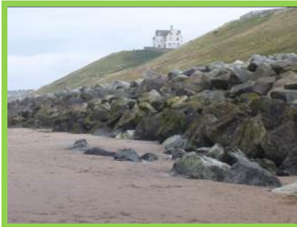
Rock revetment, promenade and coastal slopes of Whitby West Cliff (D0801C01)
