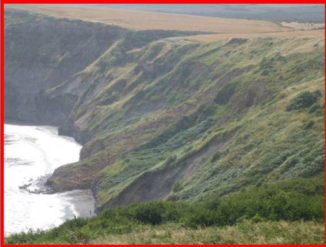
MU6/5 – View of the landslip looking across Port Mulgrave from west to east (Totally Active)
