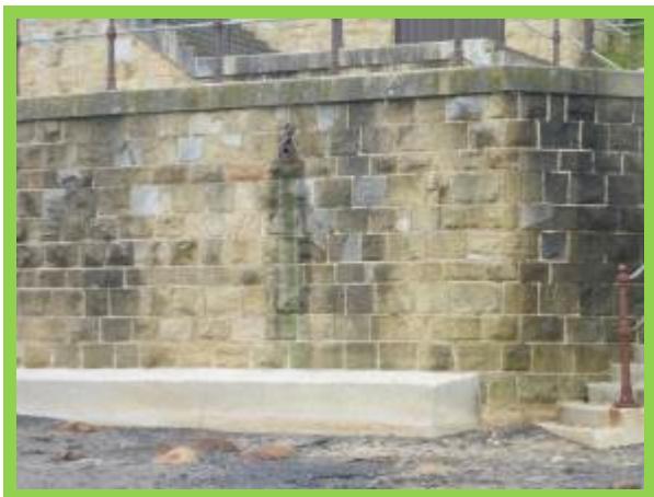
New seawall around pumping station (/1003C07)
