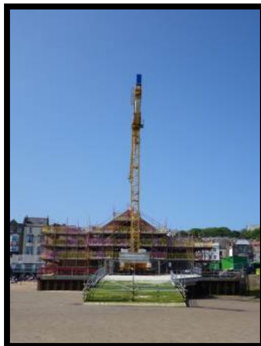
Construction of new RNLI lifeboat station and slipway (/1301C08 & C20)
