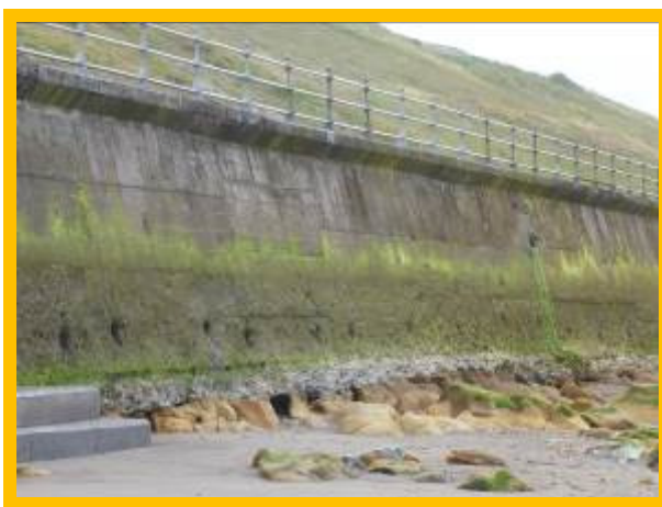
Junction between new concrete toe and original undercut toe (D0802C01)
