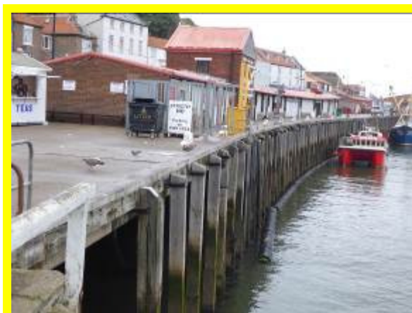
Generally fair condition of suspended deck section of quay wall (\803C06)
