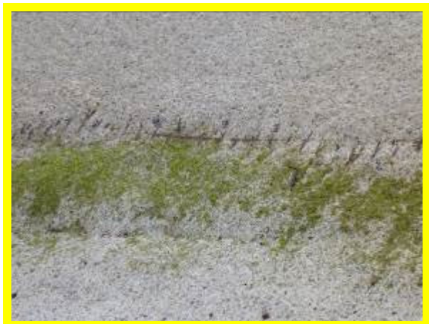
Exposed rebar (D0701C02)
