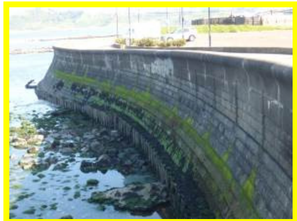
Fair condition seawall at Sea Life Centre (/1201C02)
