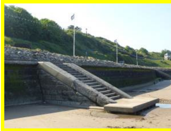
Fair condition seawall with recent repairs to access steps (/1201C24)
