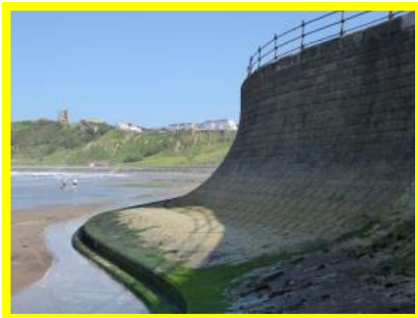
High curved-profile seawall (/1201C07)
