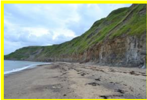
Steep mudstone cliffs with overlying shallower sloping till with local slumps. MU8/1 Locally Active in June 2016
