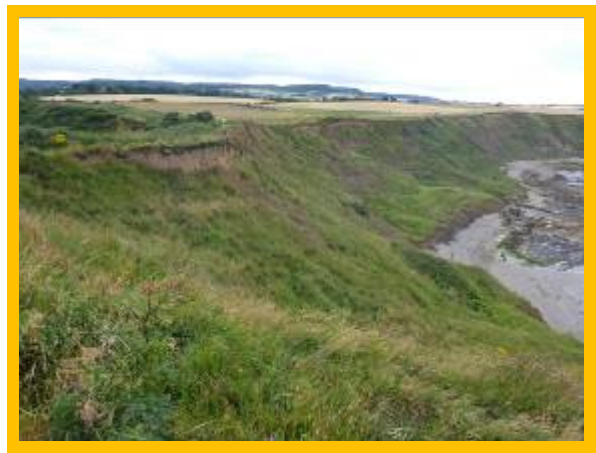
MU19/10 Landsliding (Partly Active)
