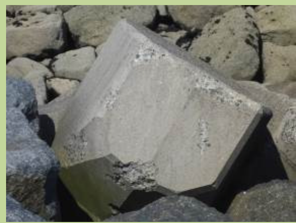
Locally abraded Accropode unit but otherwise good condition revetment (/1202C04)
