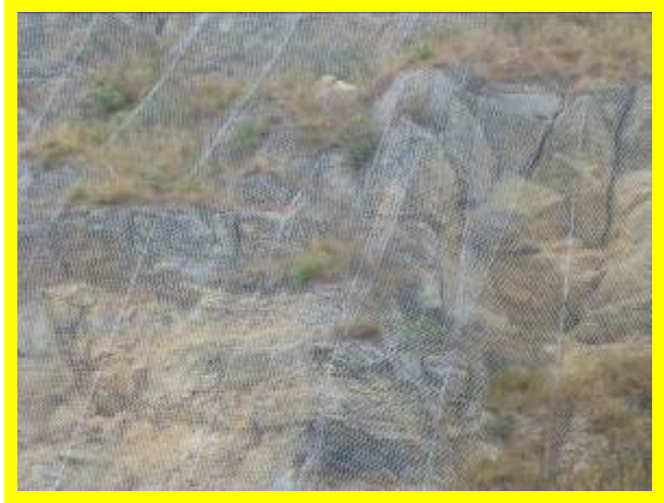
MU21/2 Rock netting on parts of Castle Headland cliff (Locally Active)
