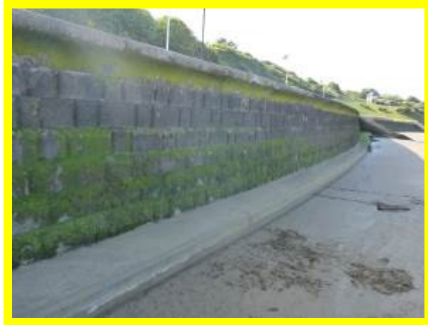
Fair condition seawall with recent repairs to toe apron (/1201C24)
