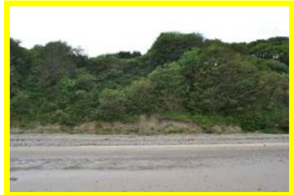
Toe of Tenants' Cliff complex. MU24/B1 Locally Active in June 2016
