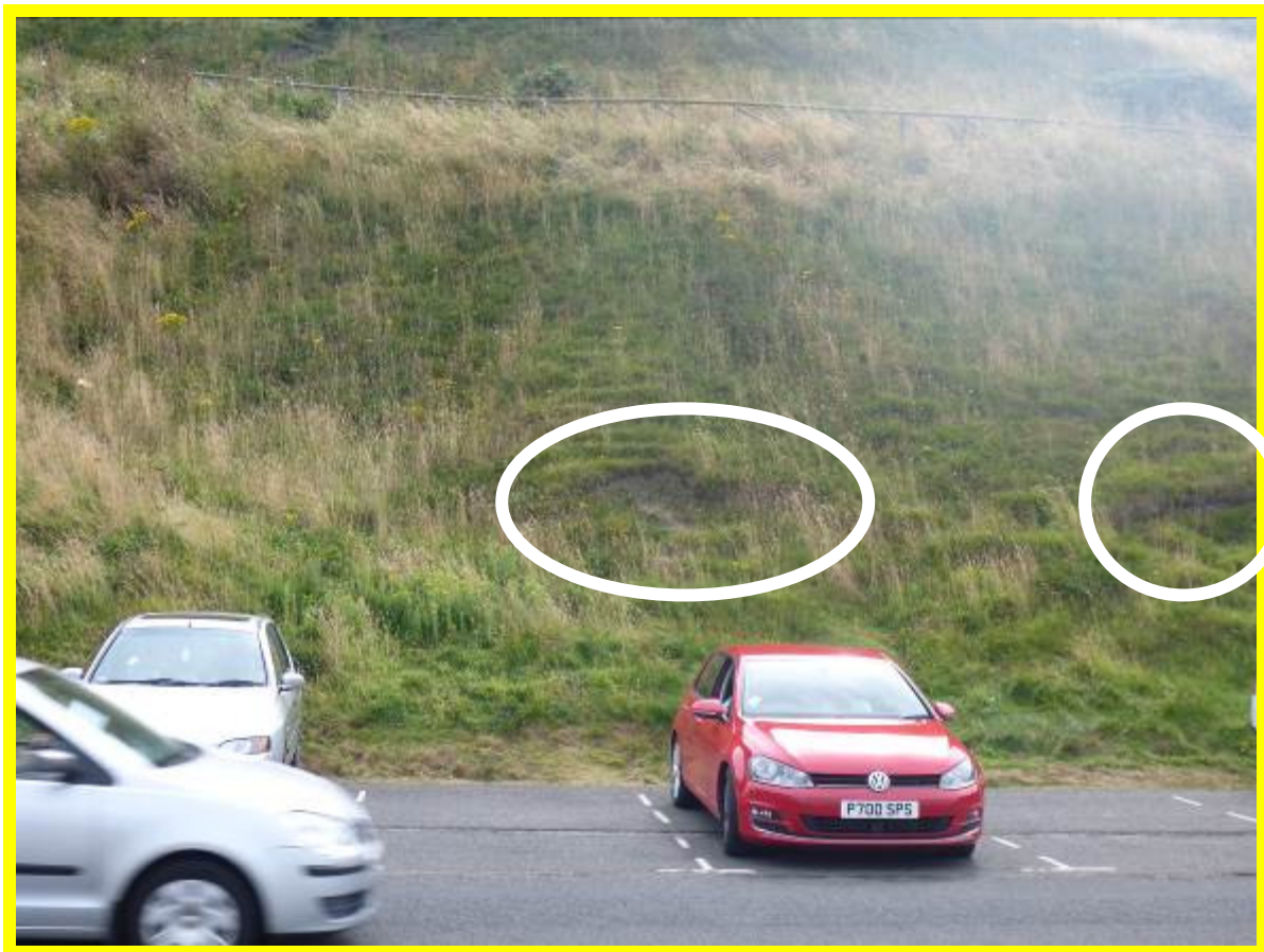
MU20/4b Cliffs in southern North Bay showing some signs of shallow slippage (Locally Active)
