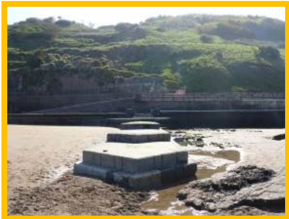
Bastion groyne in overall fair condition (/1304C02)
