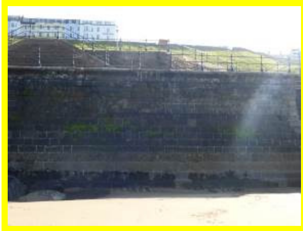
Concrete blockwall wall in fair condition (/1202C23)
