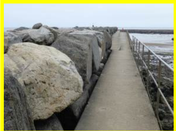
Crest blocks and deck of North Breakwater (/0402C01)
