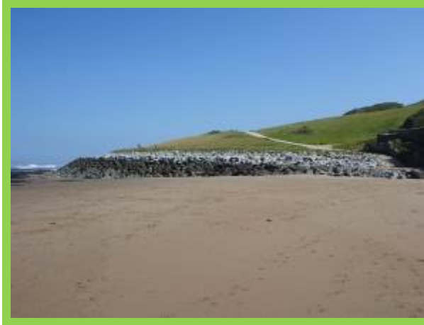
Rock revetment around debris lobe of Holbeck Hall landslide (/1304C01)
