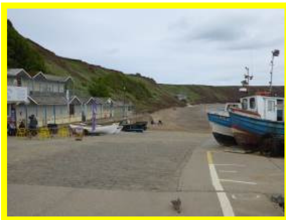
Coble Landing slipway blockwork in fair condition (/1602C01)
