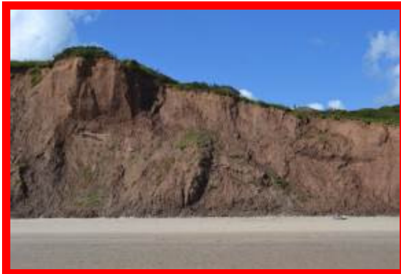
Intense erosion of till cliffs south of Hunmanby Gap. MU27/BG Totally Active in June 2016
