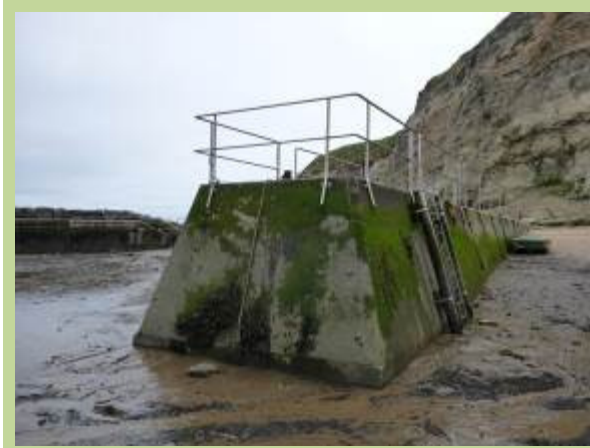
Inner harbour concrete breakwater (/0403C04)
