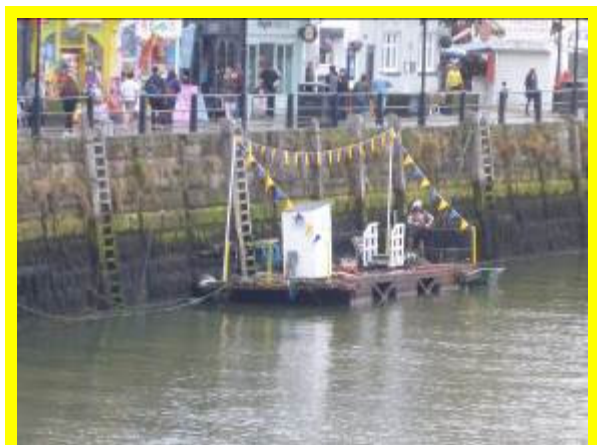
Generally fair condition of blockwork section of quay wall (\803C07)
