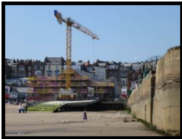
Construction of new RNLI lifeboat station and slipway (/1301C08 & C20)
