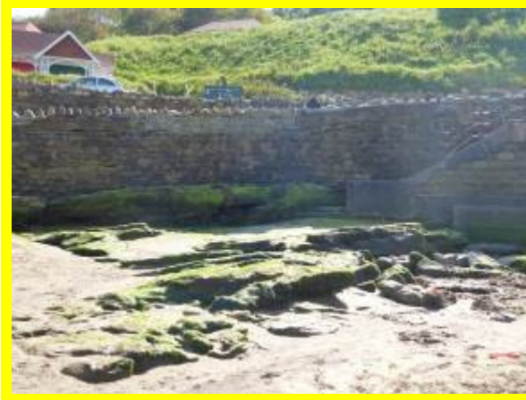
Overall fair condition of low stone wall (/1302C03)
