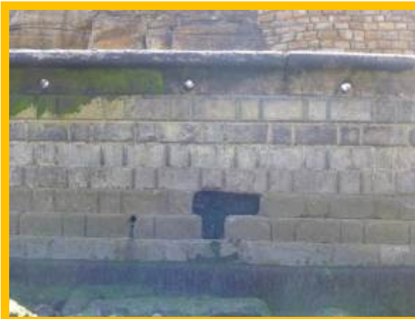
Overall fair condition of low stone wall (/1302C02)
